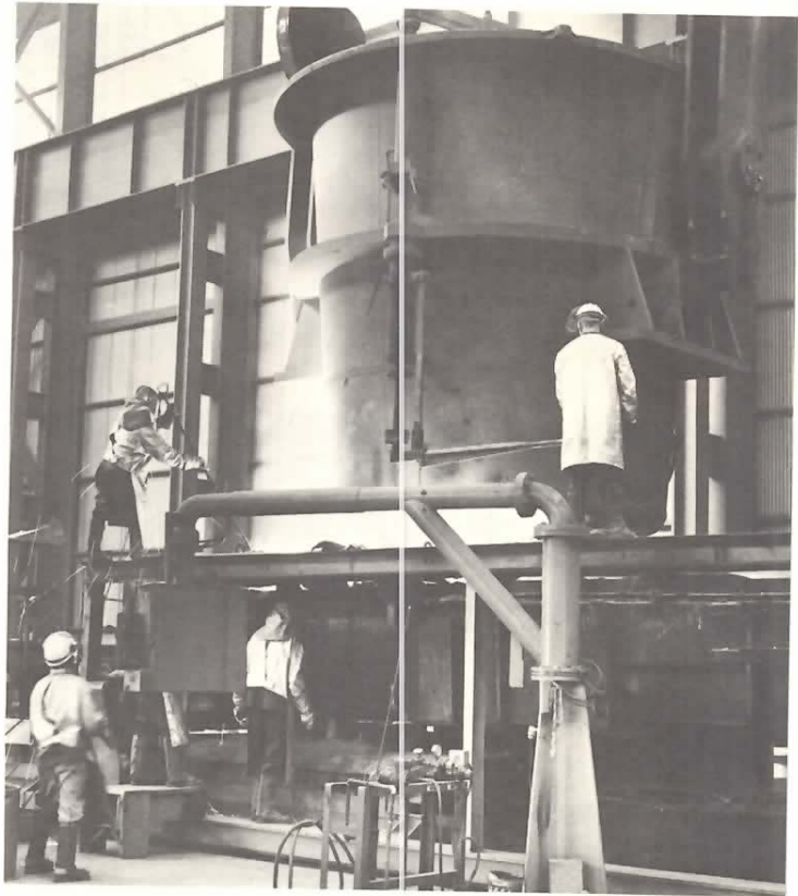
Molten steel from furnace ladle is released into tundish then passes through snorkel tube in oscillating mold (lower center) of continuous casting machine.
