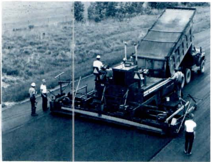
This Matmaker asphalt finisher uses a Screw Conveyor at the back of the tractor unit to move material outward in both directions and spread it uniformly across the entire paving width.
