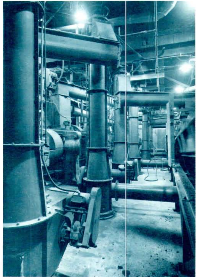
Rubber reclaiming operation uses high capacity, compact Screw-Lift and screw conveyor system to transport rubber back and forth between mills and screeners.
