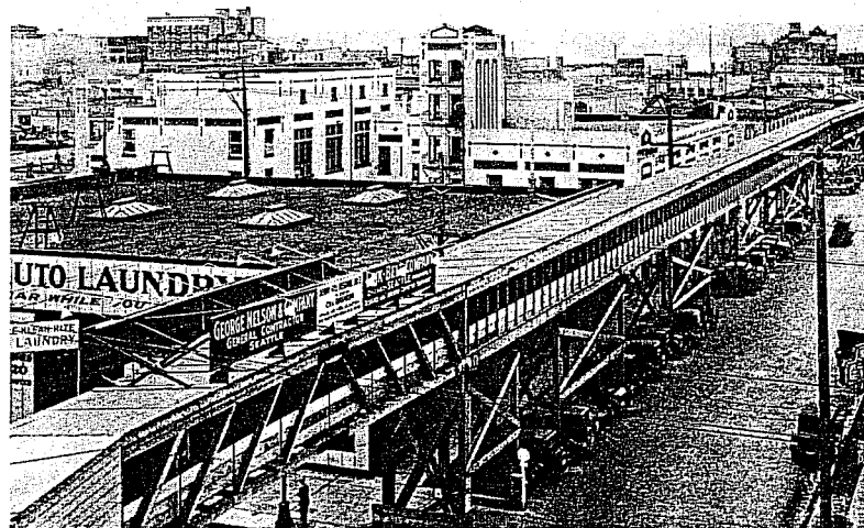
FIGURE 1.21. Denny Hill conveyor system safely moves excavated material through commercial section of city to scows in harbor.
