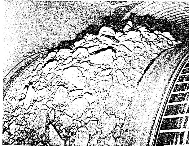
FIGURE 1.9. Material discharging over conveyor head pulley.
